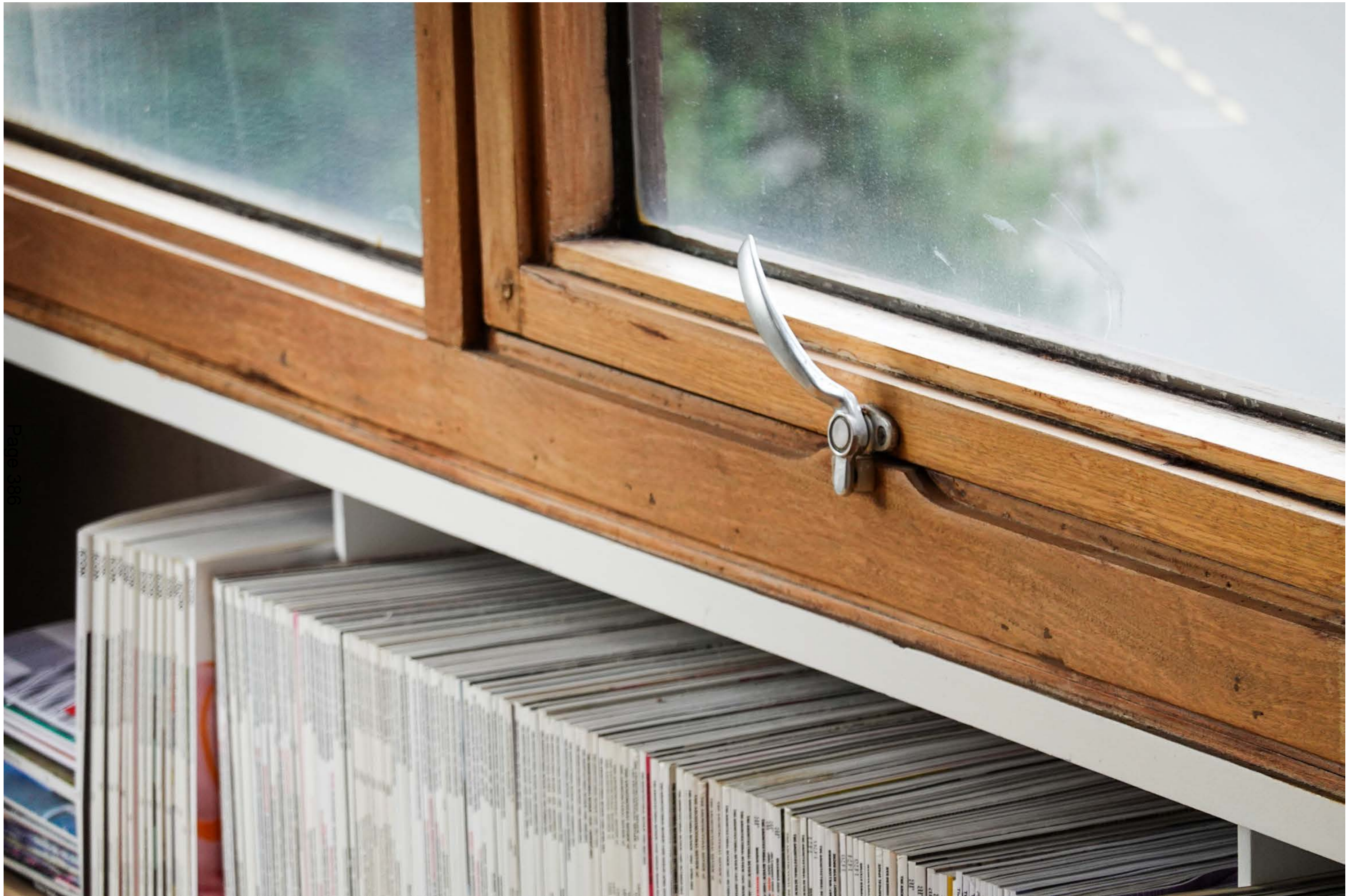
PHOTO TO SHOW QUALITY OF EXISTING JOINERY
