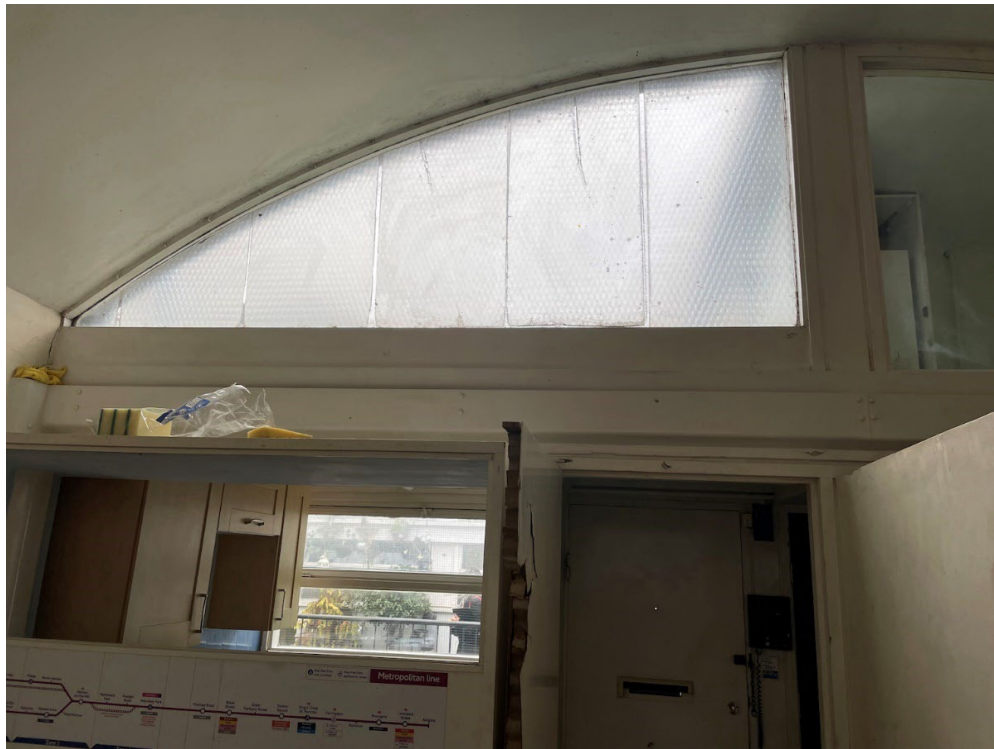
Image 8 – internal view of flat 347 vaulted window
