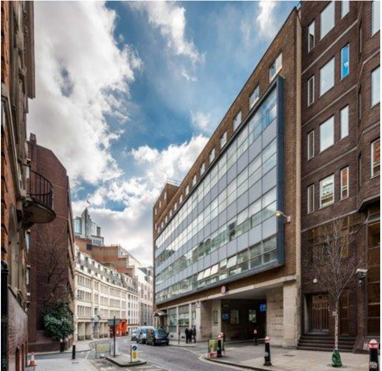
View looking south on Jewry Street
