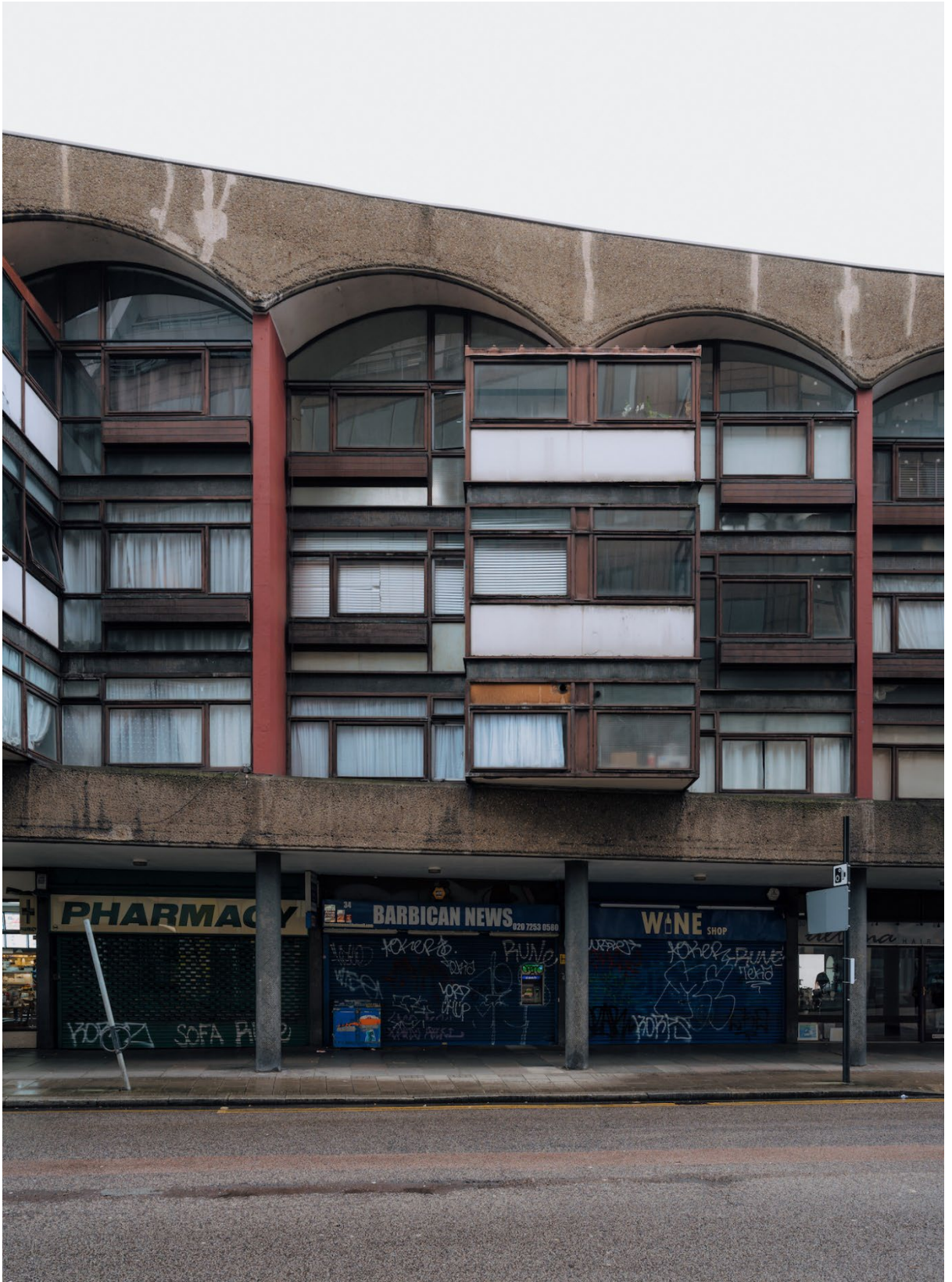
Image 1 – Crescent House, Goswell Road elevation
