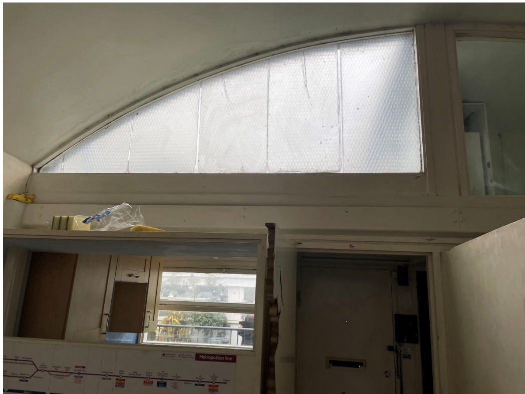
Image 8 – internal view of flat 347 vaulted window
