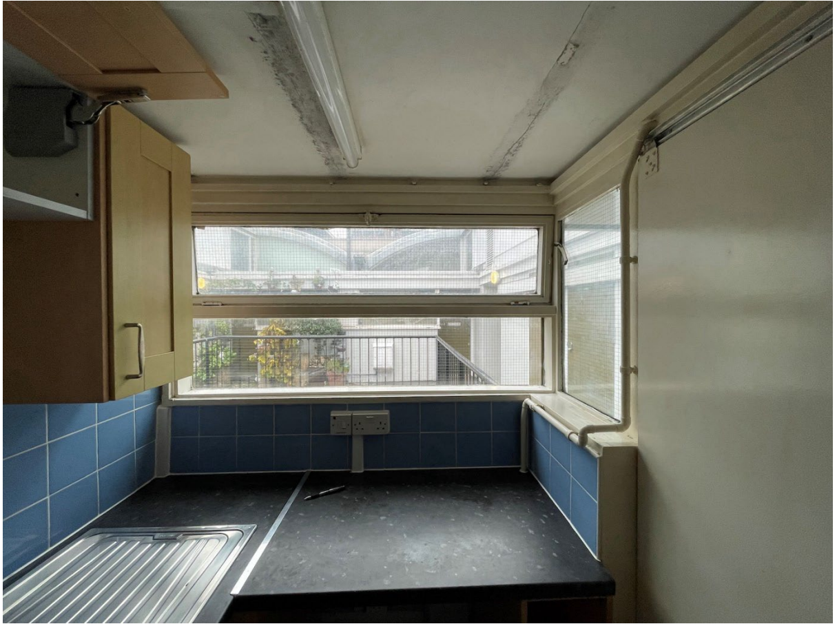
Image 7 – internal view of flat 347 lightwell windows
