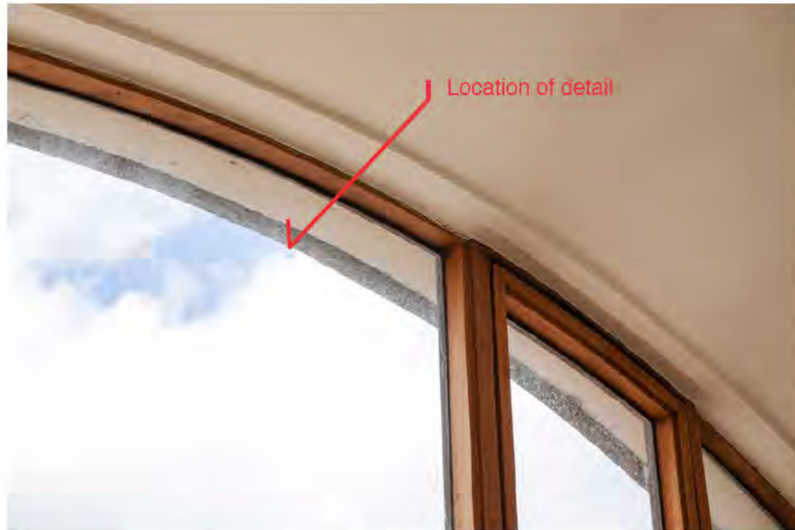
PHOTO OF EXISTING CONDITION
