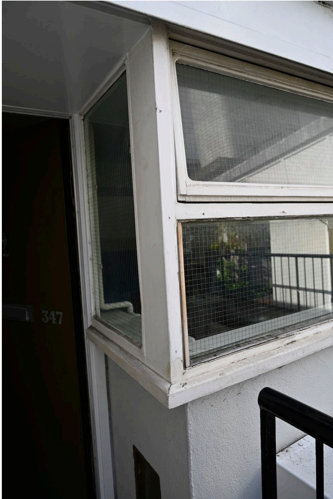
Image 5 – close up of lightwell elevation window
