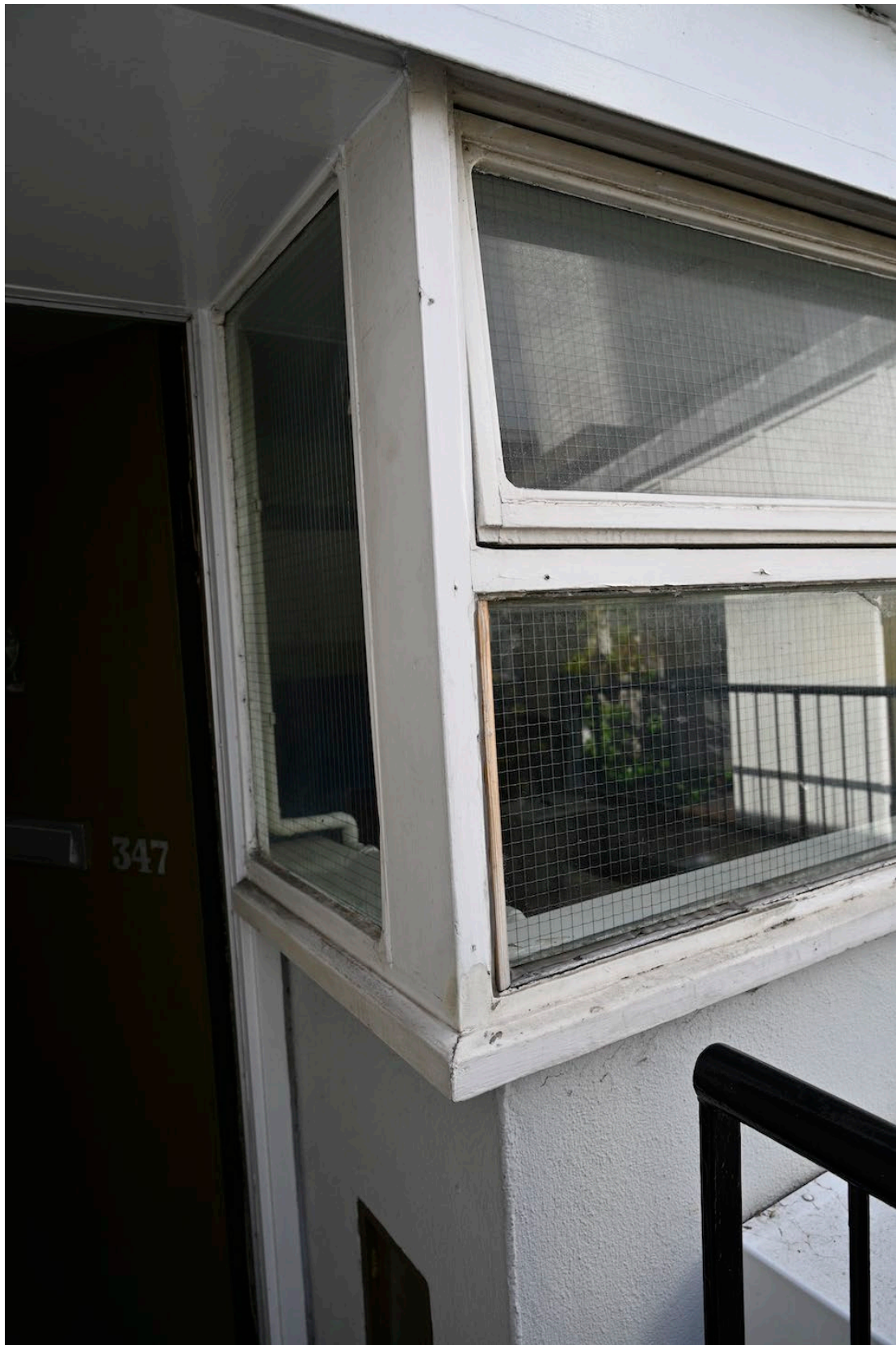
Image 5 – close up of lightwell elevation window
