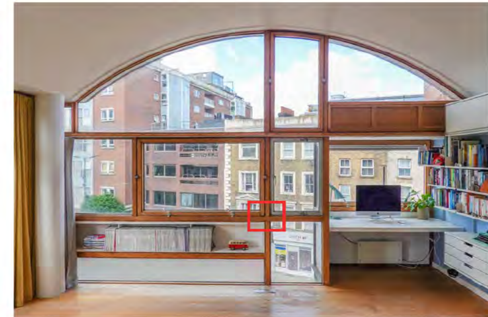
Photo showing location (EXISTING)
