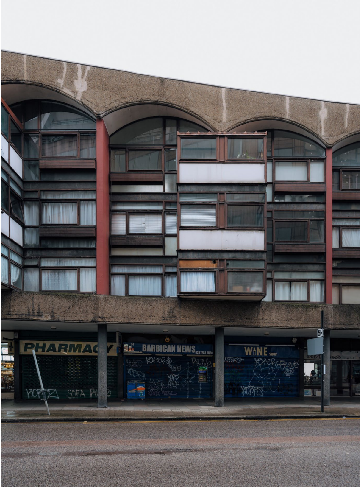
Image 1 – Crescent House, Goswell Road elevation
