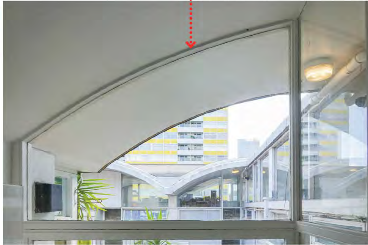
Photo showing EXISTING kitchen windows
