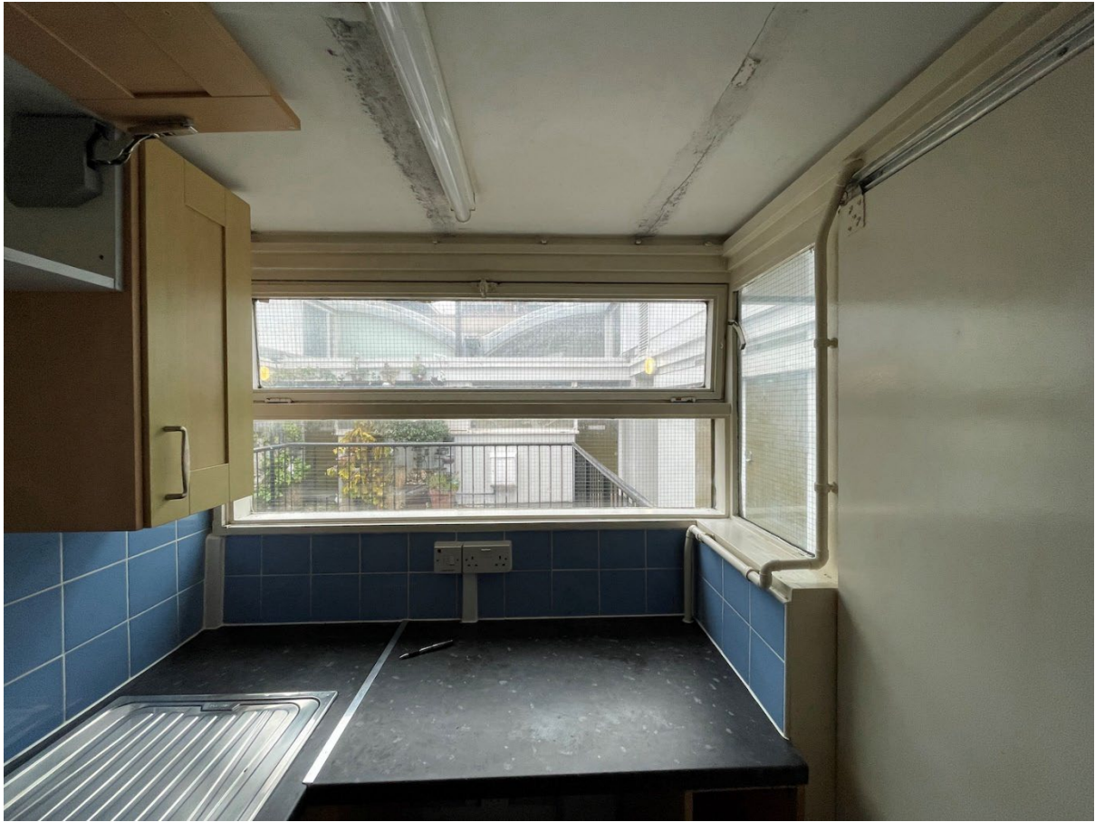
Image 7 – internal view of flat 347 lightwell windows
