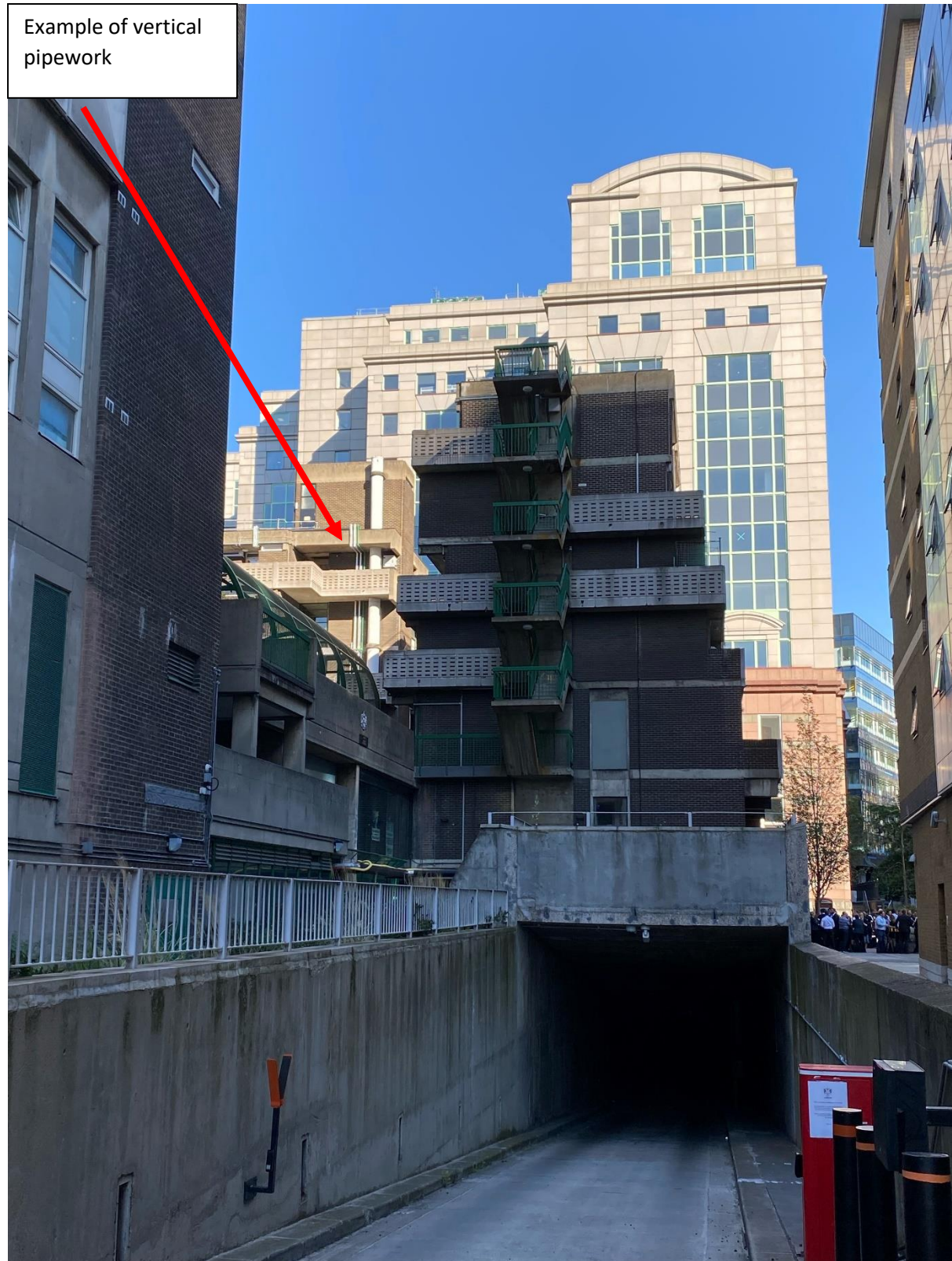
White Kennett Street Block looking south east
